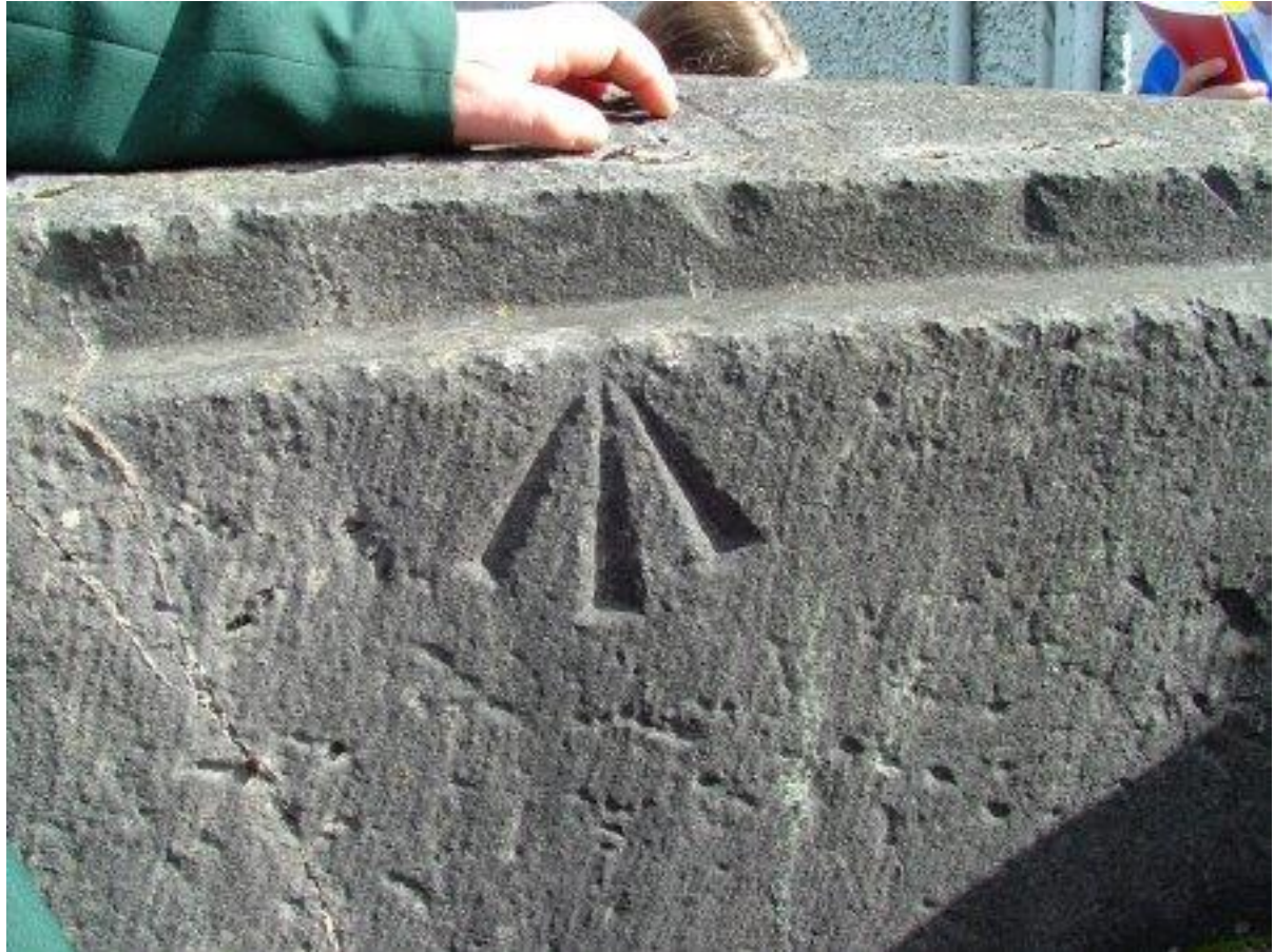
15: Sapper's Mark / Benchmark / Crow's Feet (Bridge Street)
